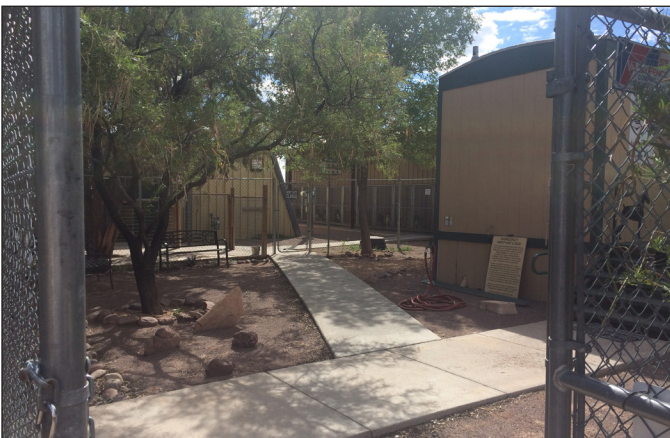
Socorro shelter as it is today looking through the front gate. Walkways lead to the office on the right and back to the original building (left) and the new larger building and outdoor kennels completed in 2003 in the background.
